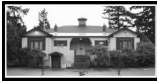
Above: Haller Lake Community Center
